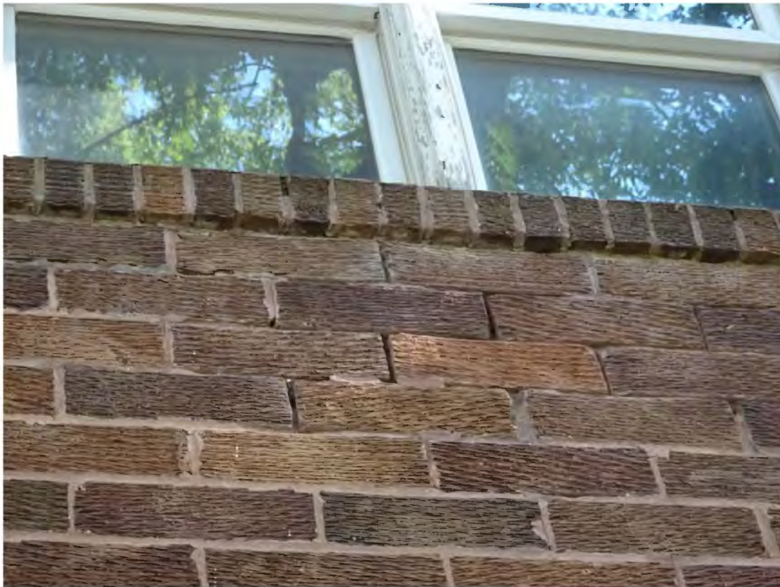
Needed Repairs – Tuck-Pointing, Window Frame Painting / Sealing
