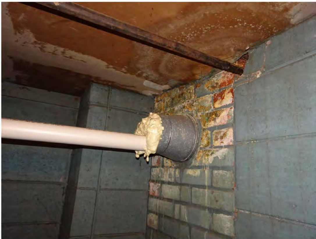
Interior View – Basement Base of Chimney Water Damage
