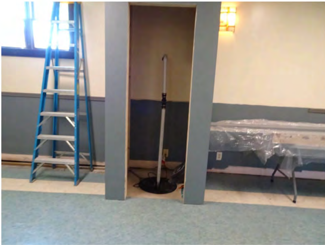
Newly Installed Sump Pump
