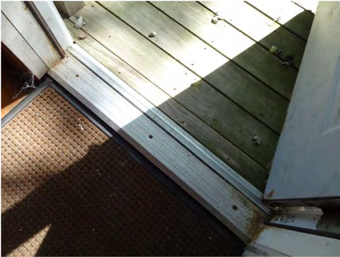
Non-Accessible Ramp Entry Threshold
