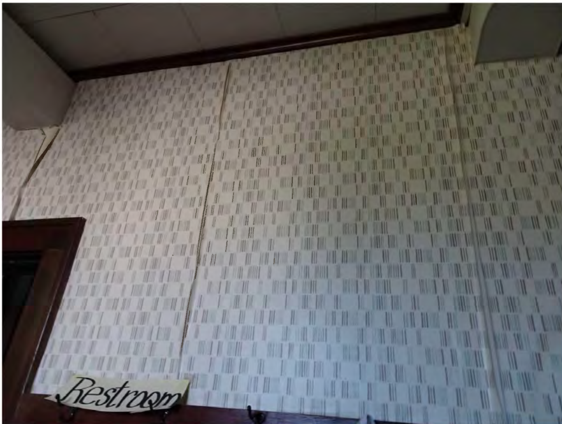
Delaminating Wallpaper
