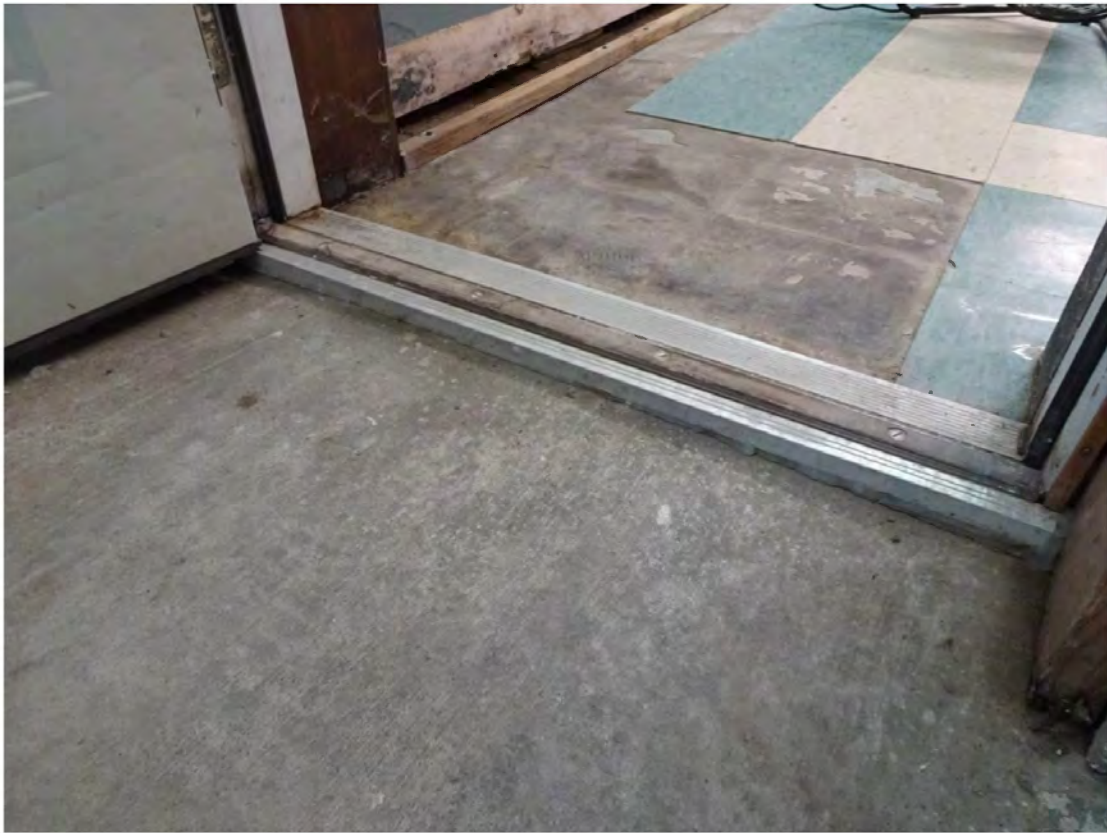
Non-Accessible Lower Level Ramp Threshold
