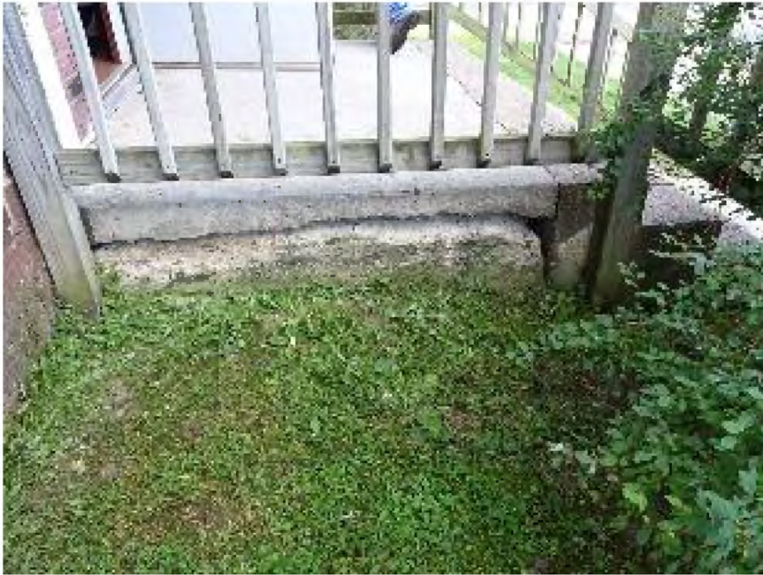
Front Stair Degradation
