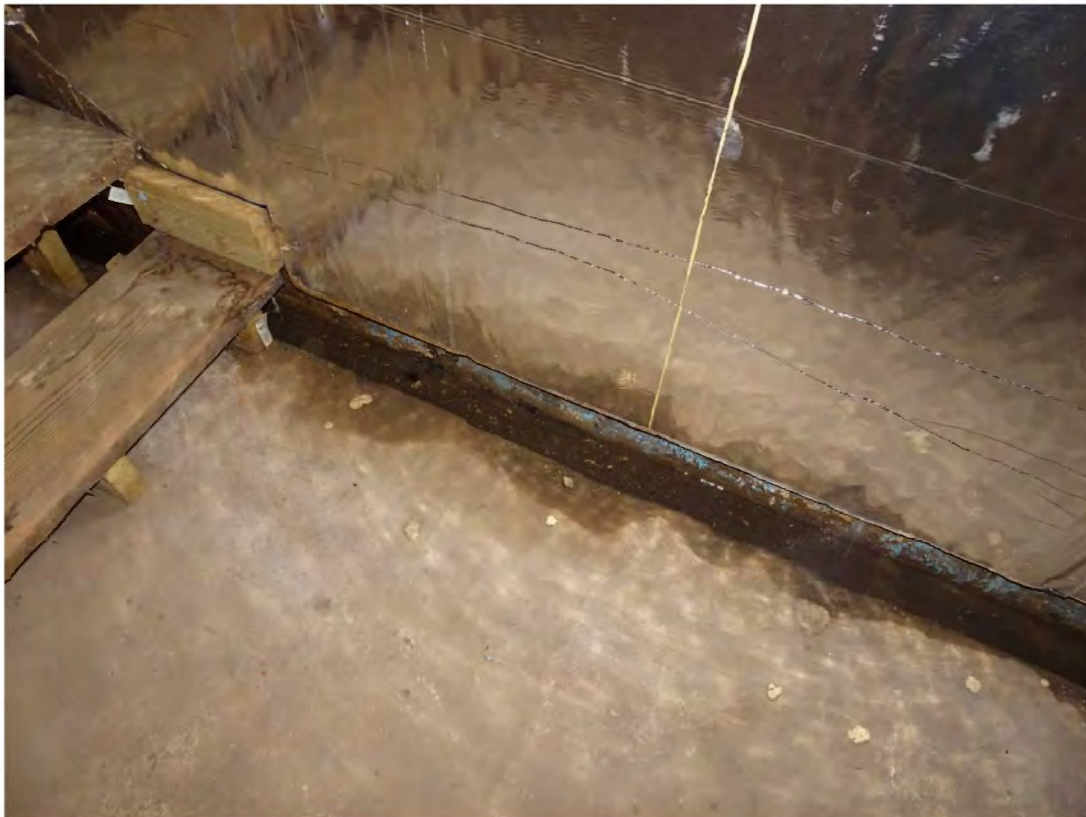
Interior View – Basement Perimeter Seepage Drainage Trench
