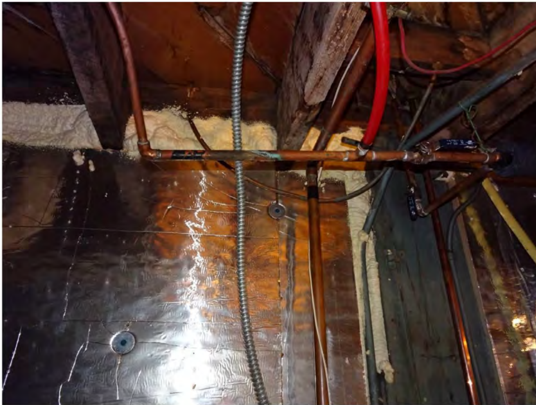
Interior View – Basement Plumbing, Spray Foam Insulation, Potential Dry Rot
